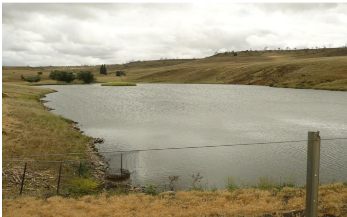
*Photo of dam at "Kydrabah"
